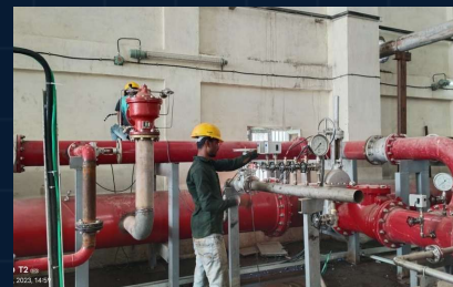
Valve station maintenance
